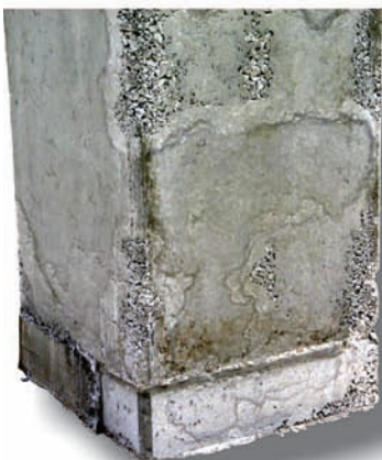
With high-cycle vibration in congested rebar
